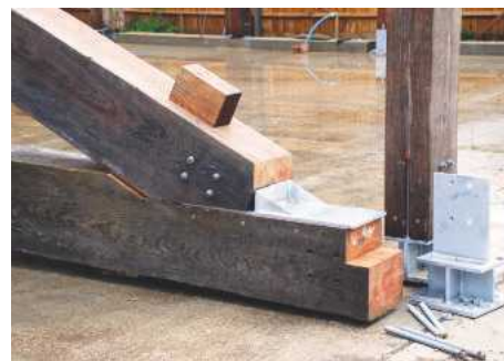
Substantial steel plates bolted to the beams enable them to be fixed securely
